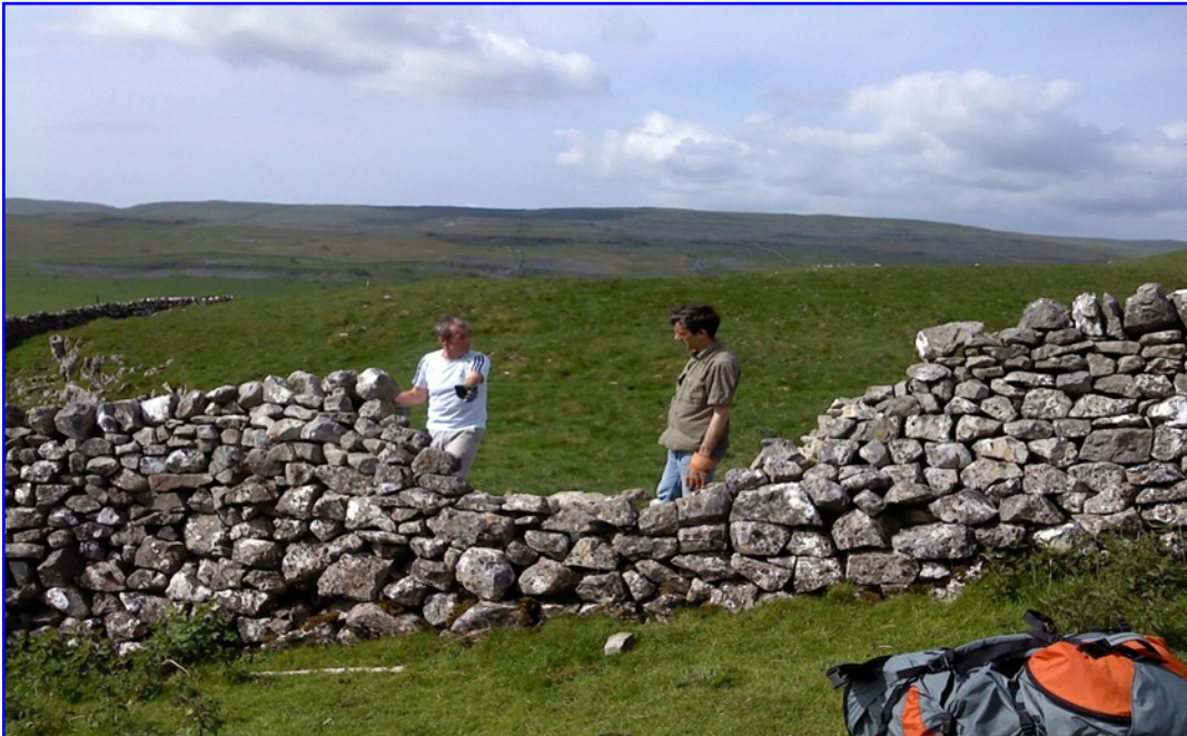
The start of a long hard day dry stone walling
